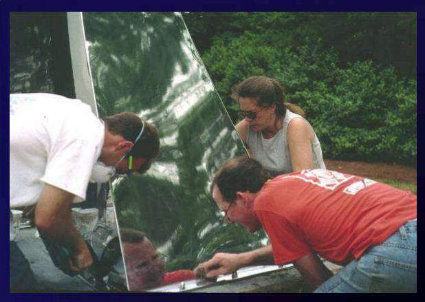
The sculpture is welded to the foundation frame and the weld is cleaned and polished.
